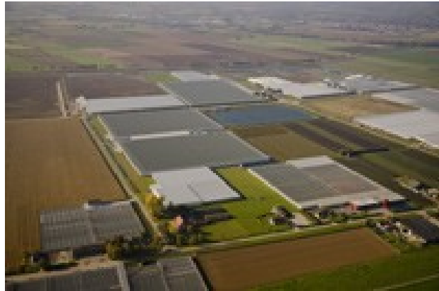
Fig. 1. Greenhouse area with total energy installations, supplying CO 2 , heat and electricity
