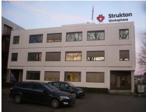
Figure 7. Testcase building in Maarsse
