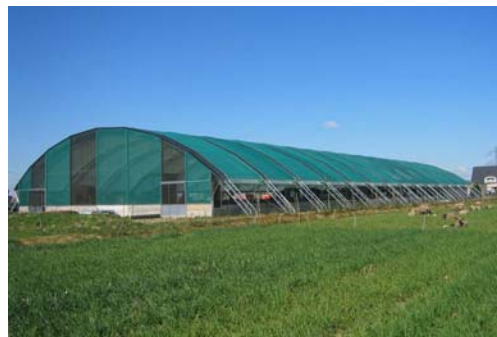
Fig 1. Pilot project arched cattle stable in Dieteren (The Netherlands)
