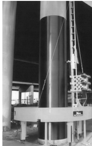
Figure 2-14: Automated FRP wrapping (fib 2001)
