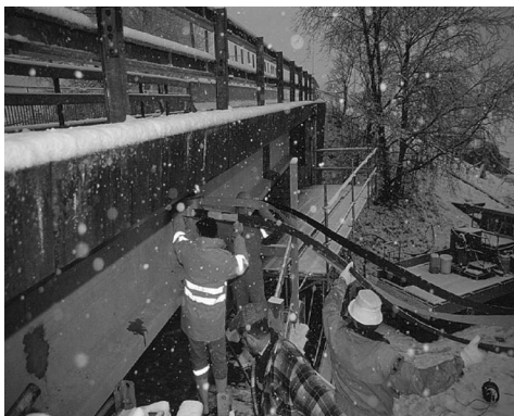
Figure 1-1: Application of CFRP laminates in cold weather conditions (Busel and White 2003)
