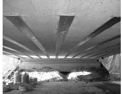
Figure 2-6: Externally bonded CFRP laminates under a bridge (Sika 2004)
