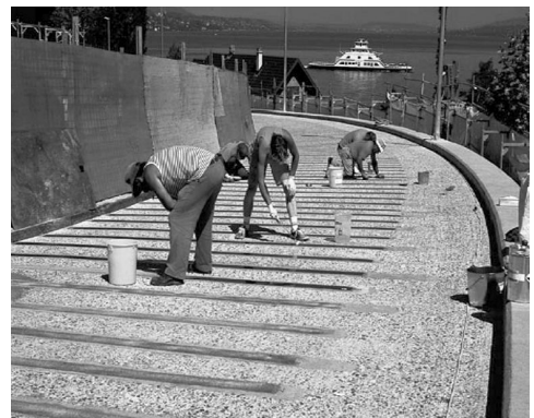
Figure 1-2: CFRP laminates that are, after applying asphalt, indirectly exposed to the sun (Busel and White 2003)
