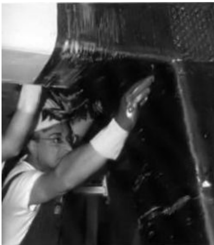
Figure 2-7: Applying the wet lay-up fabrics (Mapei 2001)
