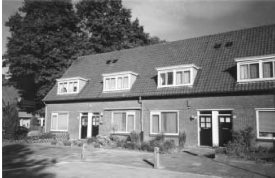
Fig. 3. Housing complex under renovation (Photo Erkelens)
