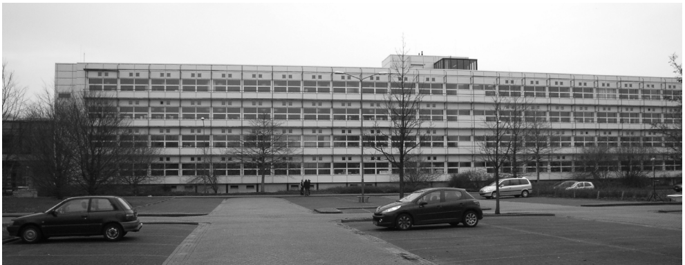
Fig. 7.12: Photo of the illuminated face of building TR.
