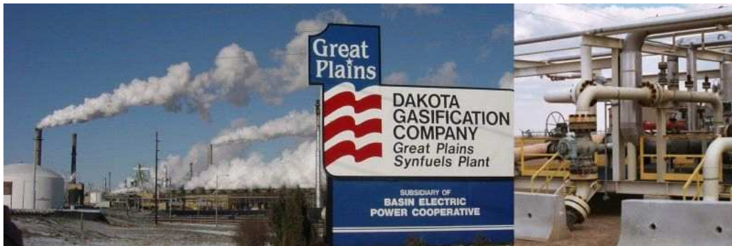
Figure 3-3: Pictures of Great Plains Synfuels plant.
