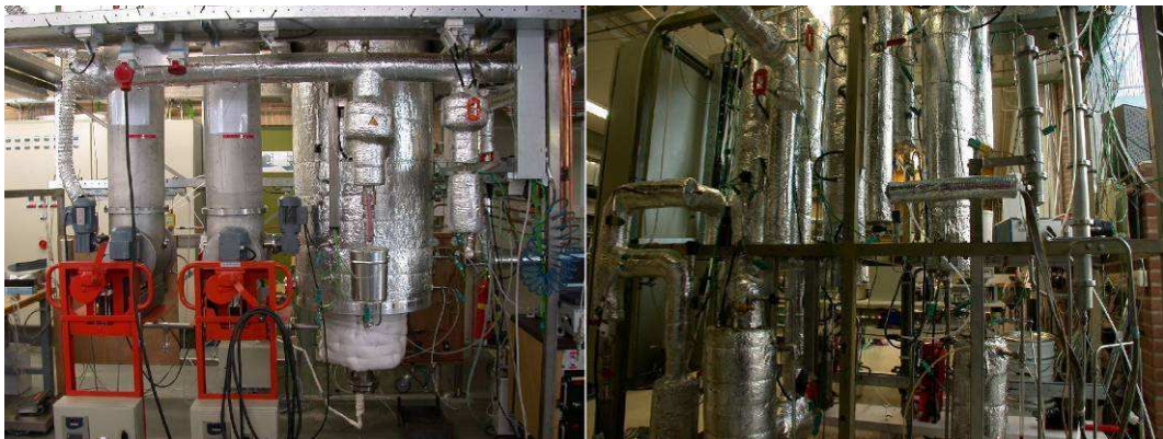
Figure 6-7: Photos of lab-scale MILENA (left) and OLGA (right) installation.
