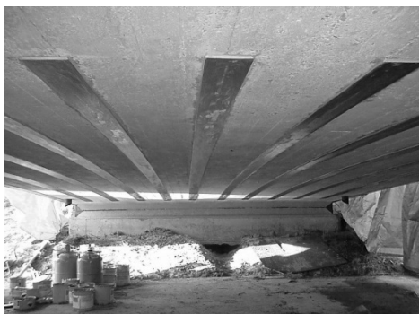
Prefabricated FRP laminates at Denekamp [Sika 2004]
