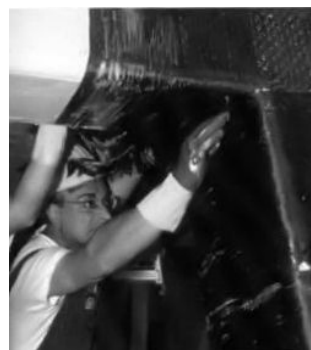
FRP fabrics for the wet lay-up system [Mapei 2001]
