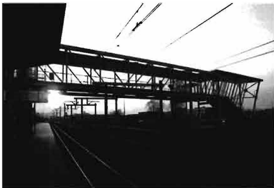
Fig. 1 Typical footbridge near a train station (Boxtel, The Netherlands).
