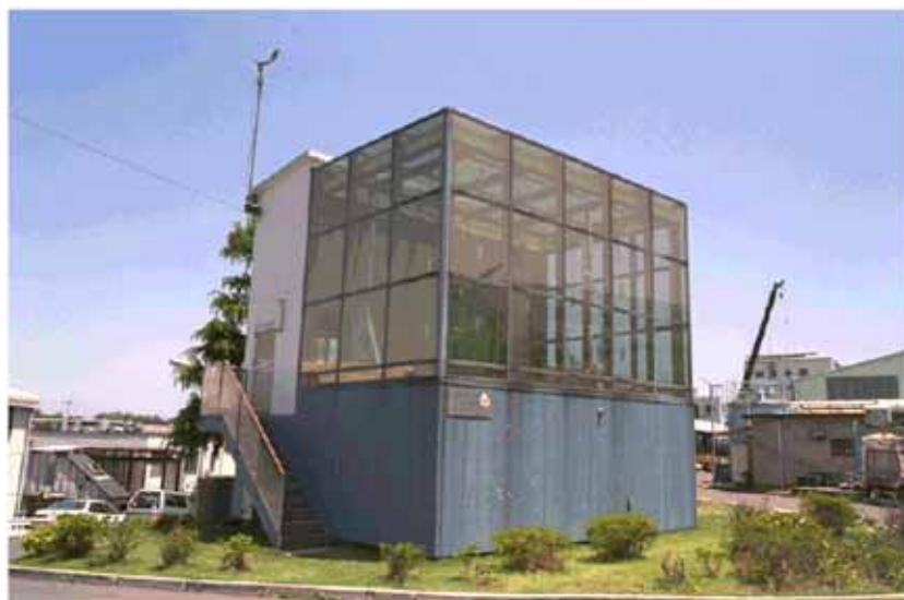
Figure 5.16 IEA Annex 26 Atrium (Yokohama, Japan)
