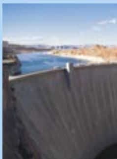
Cover photo Dam at Grand Canyon, USA © PhotoDisc
