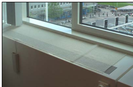
Figure 5.6 Windowsill with a (too) strong reflection coefficient is covered with material by the users
