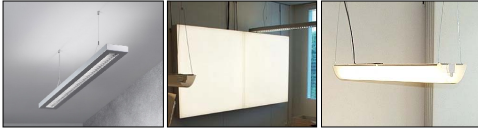
Figure 4.7 General lighting (suspended luminaire-left), large luminous area (middle) and small luminous area (right)
