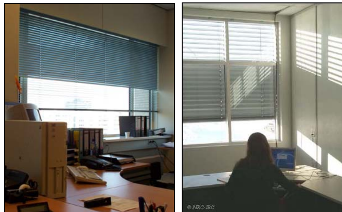
Figure 5.8 Examples of daylight control devices with adjustable zones (on the left: inside system, on the right: outside system, photo by the NRC-IRC)
