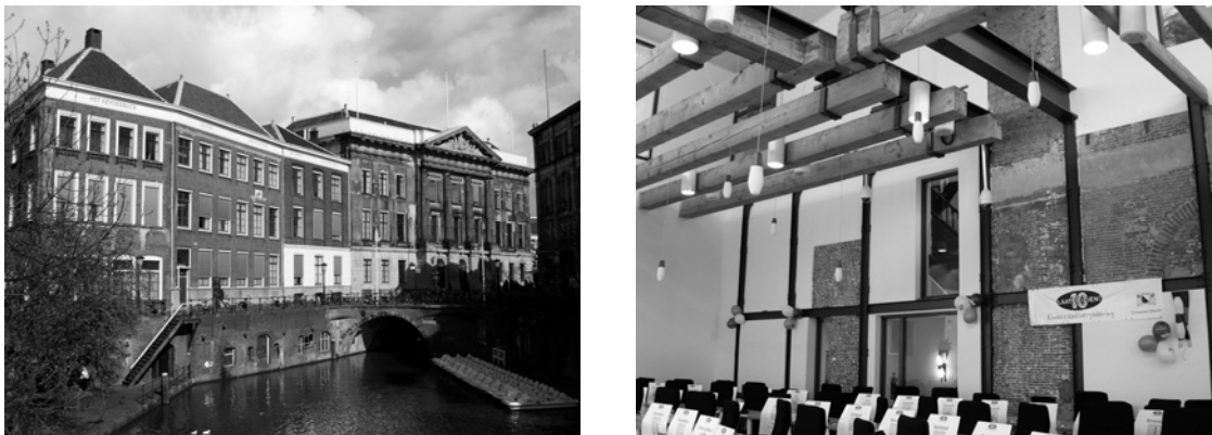
Figure 1 - Renovation of the town hall of Utrecht – the Netherlands, Enric Miralles e Benedetta Tagliabue (1996 – 1999)
