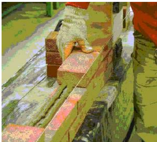
Figure 8 a) Brick laying using thin layer mortar. b) Vertical section over a thin layer mortar joint, recessed at the right hand side.
