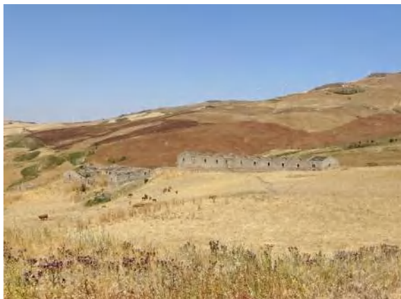
Fig. 2. Example of rural architecture (masseria) in the inner Madonie mountain area of Sicily (photo by the author).
