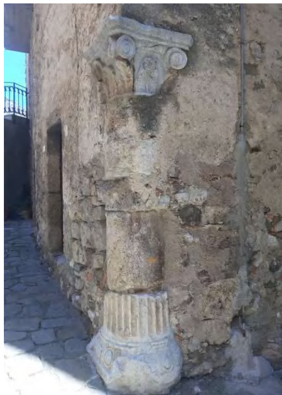
Fig. 5. Alcara li Fusi, fragments of a column and a capital (possibly ancient ones), reused in a corner (photo by A. Antista).
