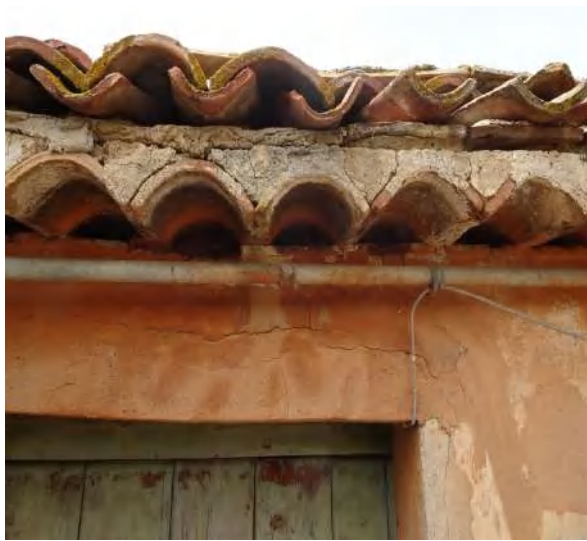
Fig. 8. Traditional construction systems, sometimes simple and necessary of a compatible technological check (photo by the author).
