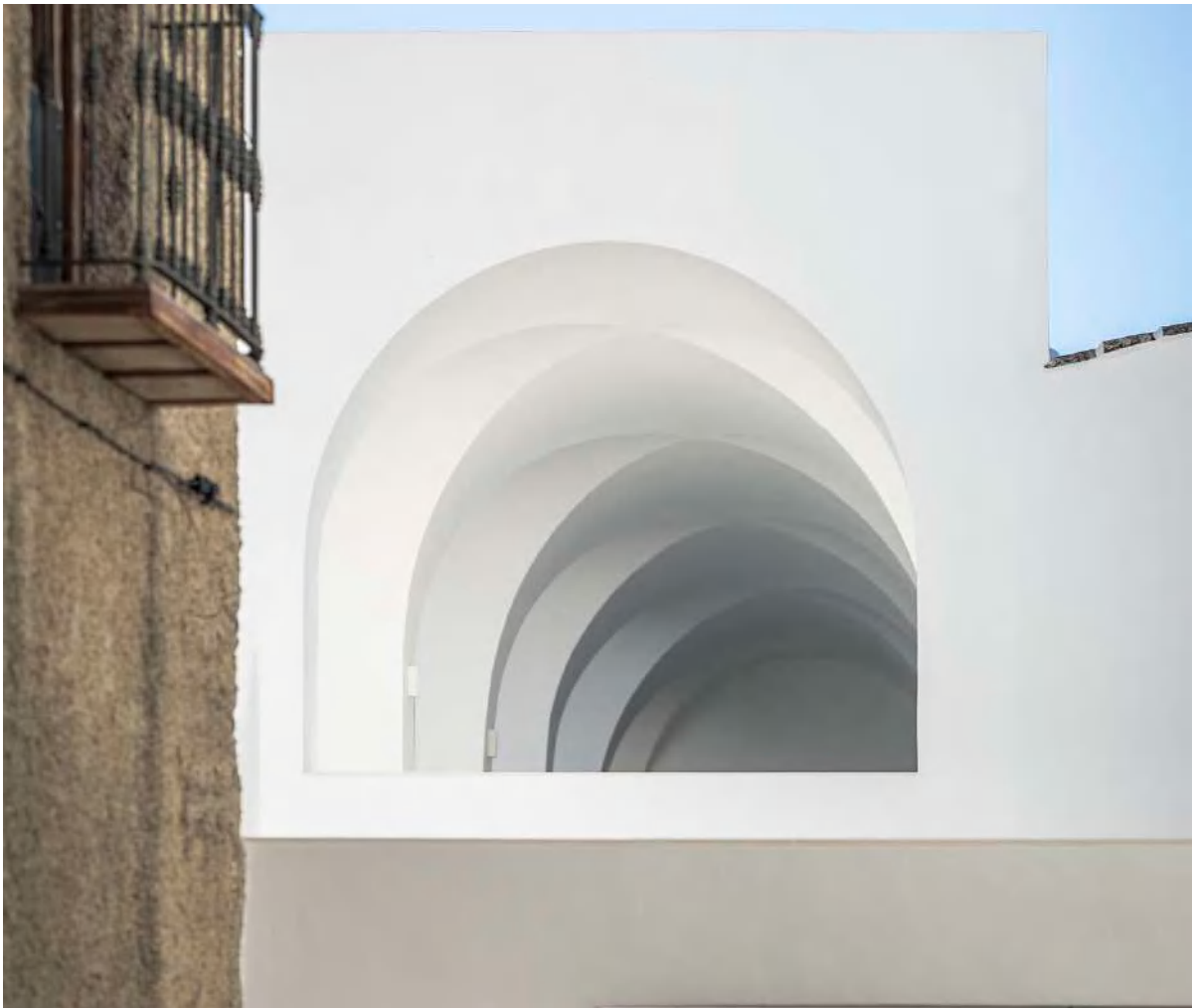
Fig. 8. Detail of the intervention.
