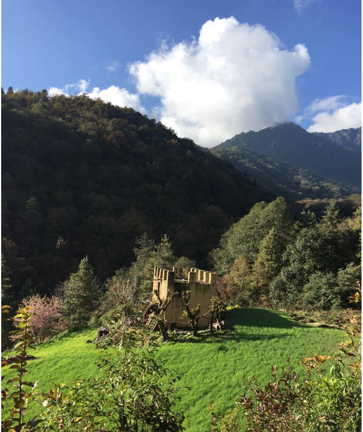
Abandoned house in the middle of the forests, on the way to one of our survey plots
