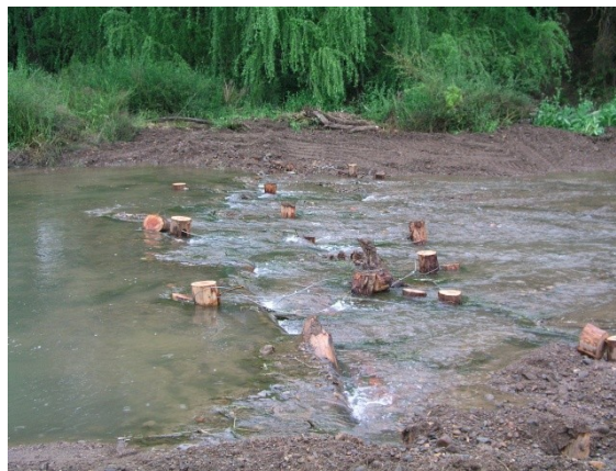
Plate 2.5 The finished log sill immediately after the dam was removed. Note that about 10 cm of the log sill is above the river bed. The wetted channel is 10 m wide.
