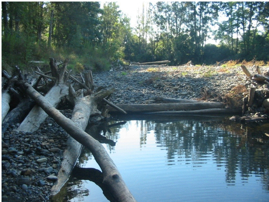
Plate 2.7 After the March 2004 flood in the Williams River, surface flow at WUM was down the left channel (to the right of the photo), dewatering the right channel. The photo was taken looking upstream with the downstream log sill in the foreground. The broken upstream log sill can be seen in the background.
