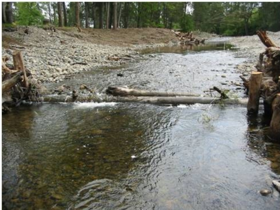
Plate 2.2 Native gravel was used to backfill the log structures. The photo was taken looking upstream from below the second (downstream) log sill.
