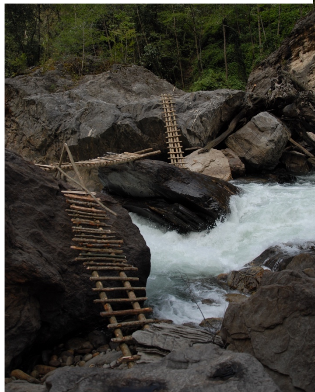
Picture: 2 A bridge constructed to access takin winter habitat at Kabina, Jigme Dorji National Park, Bhutan.
