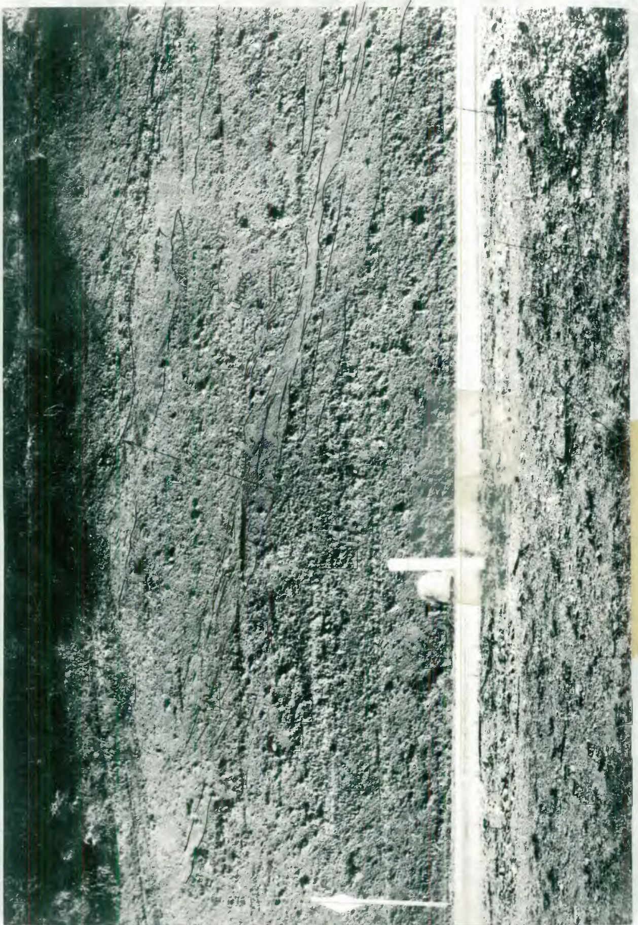
Plate 29 Early form of the Whitfield - Whitlands upper road cutting
