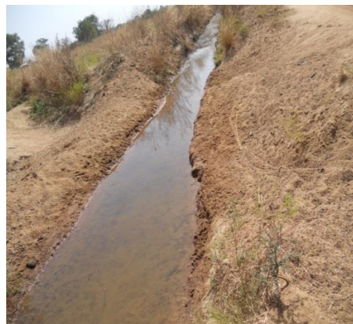
Canal with concrete walls removed, Vea
