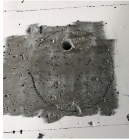
Figure 4-18: Identification of cutting area and cable passage hole.
