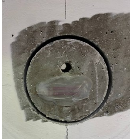
Figure 4-28: Example of SGs gluing on a low-porous surface.
