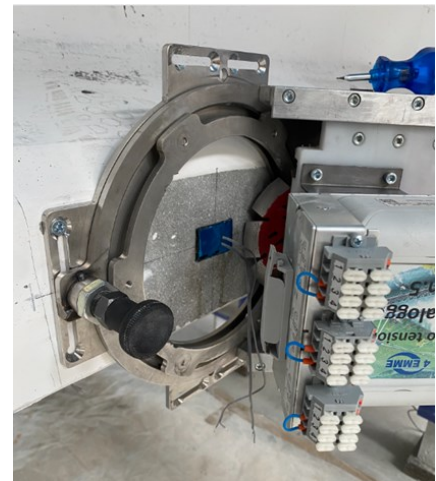
Figure 4-39: Equipment installation before vertical cutting.
