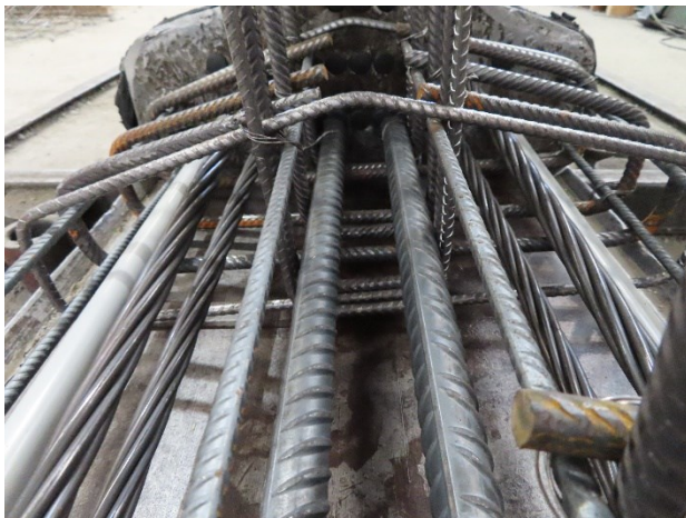
Figure 3-10: Reinforcement detail of Beam B in the factory before casting.
