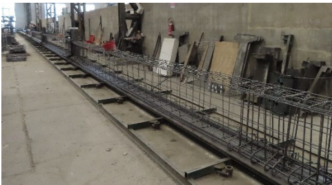
Figure 3-15: Reinforcement cage of all beams.
