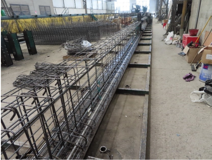
Figure 3-9: Reinforcement in the factory before casting – Beam B.
