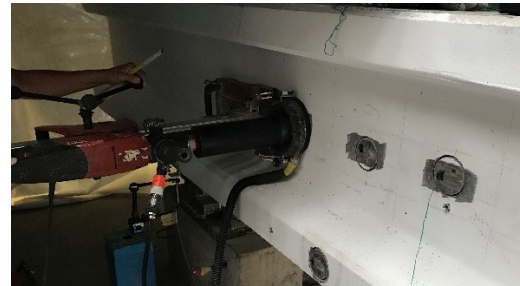
Figure 4-21: Performing the test with a wet core drill (Beam A).
