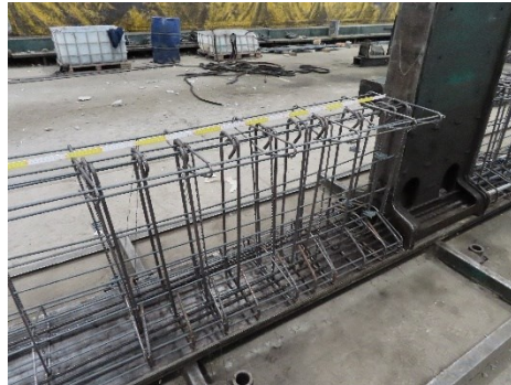
Figure 3-3: Rectangular \varnothing 12/150 mm stirrups with \varnothing 8/300 mm stirrups shaped like the "I" section in the end D-regions.
