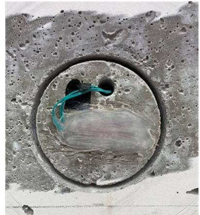
Figure 4-29: Example of SGs gluing on a very porous surface.
