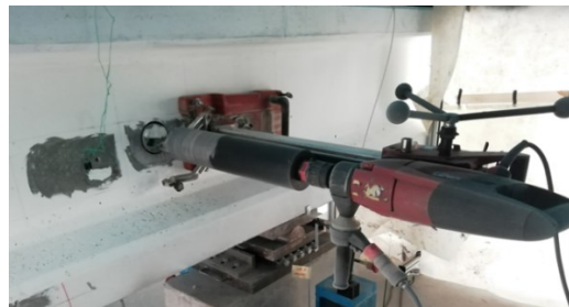
Figure 4-22: Instrumentation used to carry out concrete cores.
