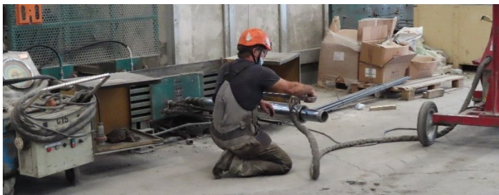
Figure 3-19: Strand tensioning phases in the factory.
