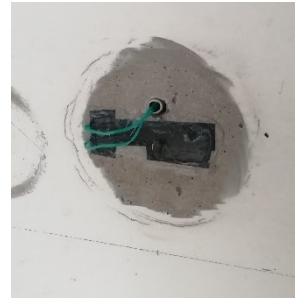
Figure 4-19: Gluing and protecting SGs from water using silicone
