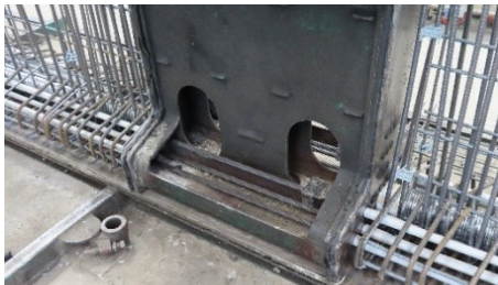
Figure 3-17: Intermediate beam formwork element for strand continuity.
