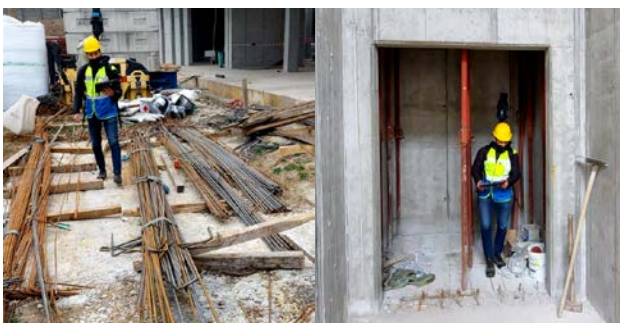
Figure 4. Mapping the construction site with the iMMS.
