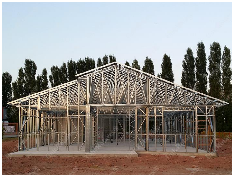
Figure 1: LSF Construction
