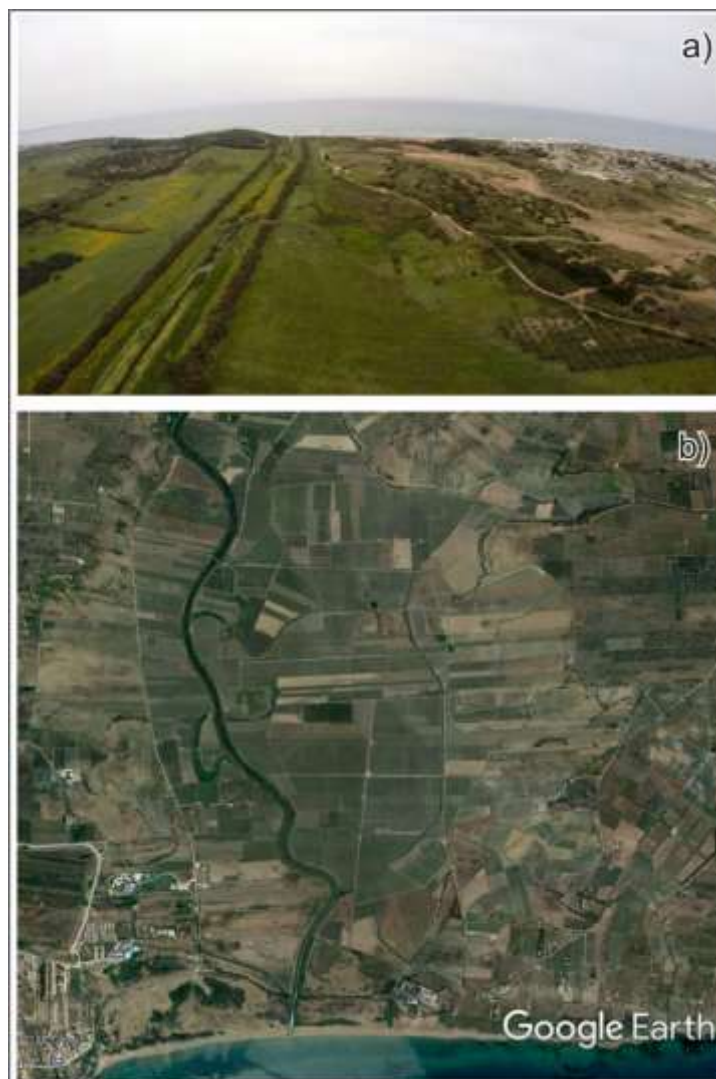
Figure 6 – a) Aerial view (from north) of the final sector of the Modione river, strongly restricted and rectified by human activities; b) satellite image (Google Earth) of the final sector of the Belice river
