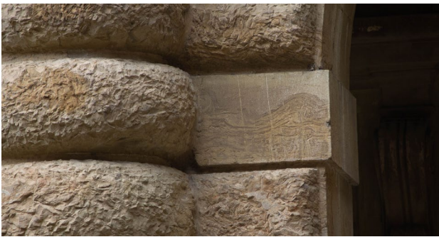
Figure 1. Detail of the convoluted lamination on the impost ashlar of the Doric order arch (August 2020).
