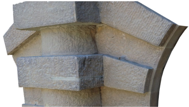
Figure 7. High-resolution textured 3D model of a detail: in addition to the stonework traces, connections between blocks, cracks, and metal elements are also visible.
