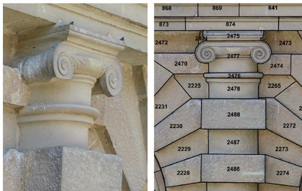
Figure 9. The capital consists of three different blocks (detail of the ortho-mosaic with identification of the blocks 2475, 2476, 2477).
