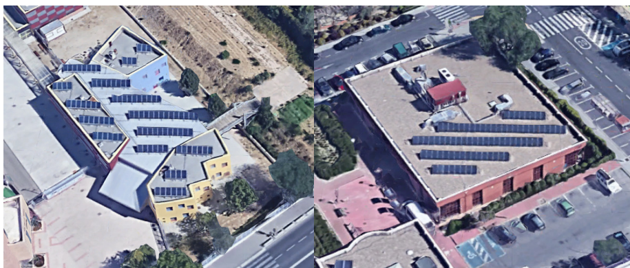
Figure 21. PV panels oriented to the south [22].
