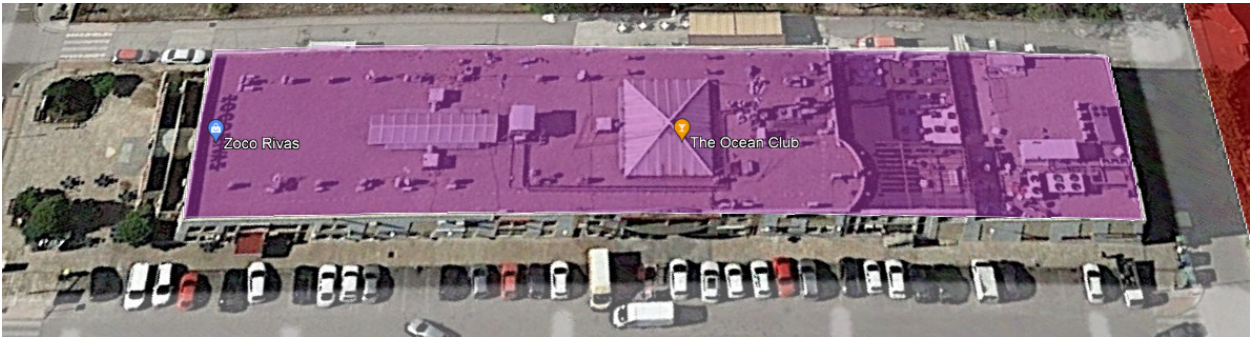
Figure 8. Zoco Rivas commercial building [9].
