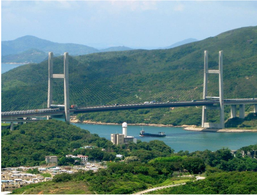
Figure 6 Kap Shui Mun Bridge[18]
