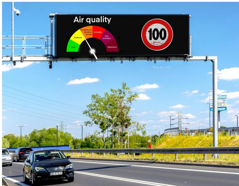
Figure 31 Schematic visualisation of VMS used in the bridge [63]
