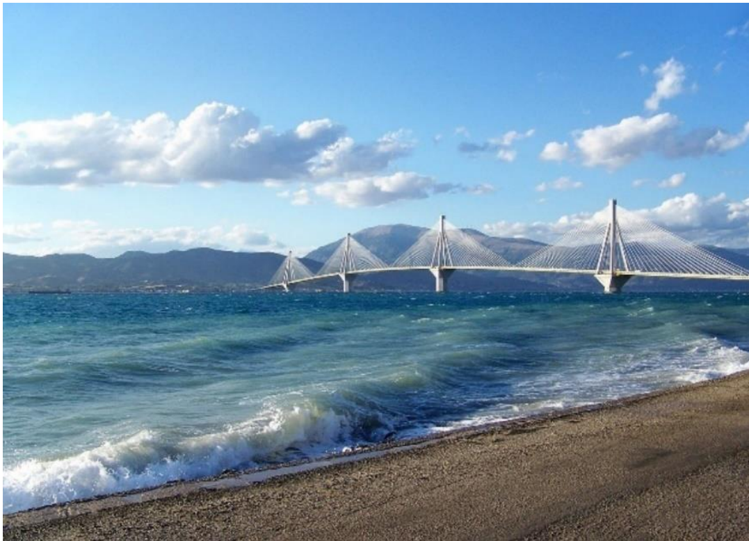
Figure 4 The Rio- Antirro Bridge[16]
