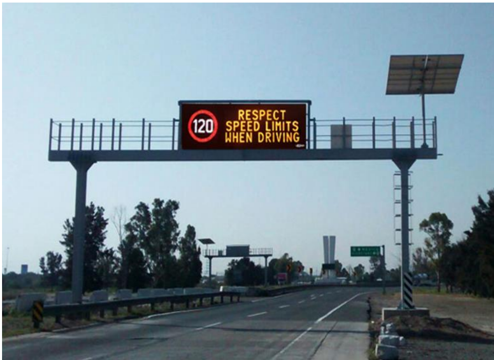
Figure 30 Example of VMS[62]
