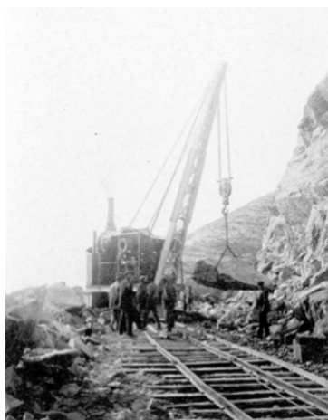
Figure3 :Construction of the road
