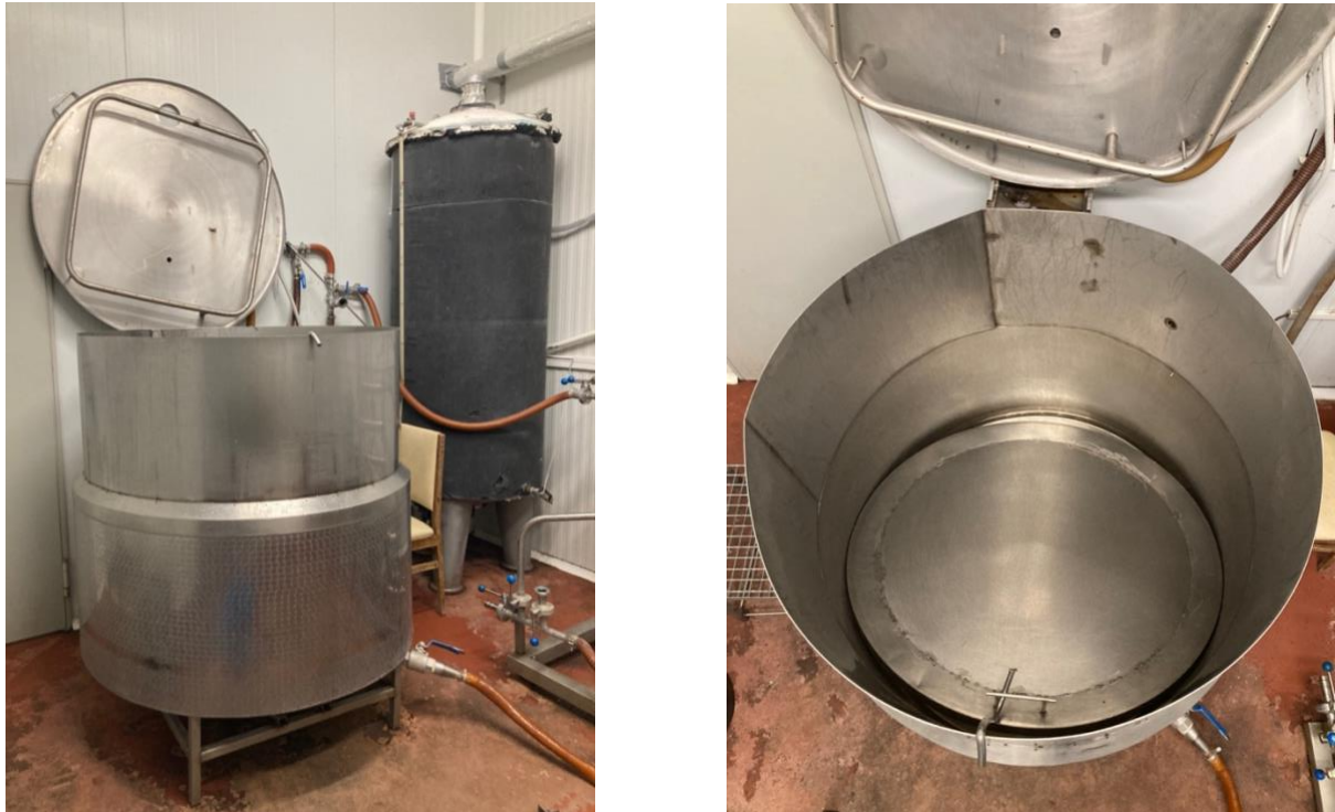
Figure 3.1 & 3.2. Heating deposit and mash tune with the filtering membrane
