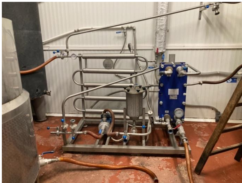
Figure 3.3. Motor used to pump the wort into the recirculation circuit, also seen in the picture
