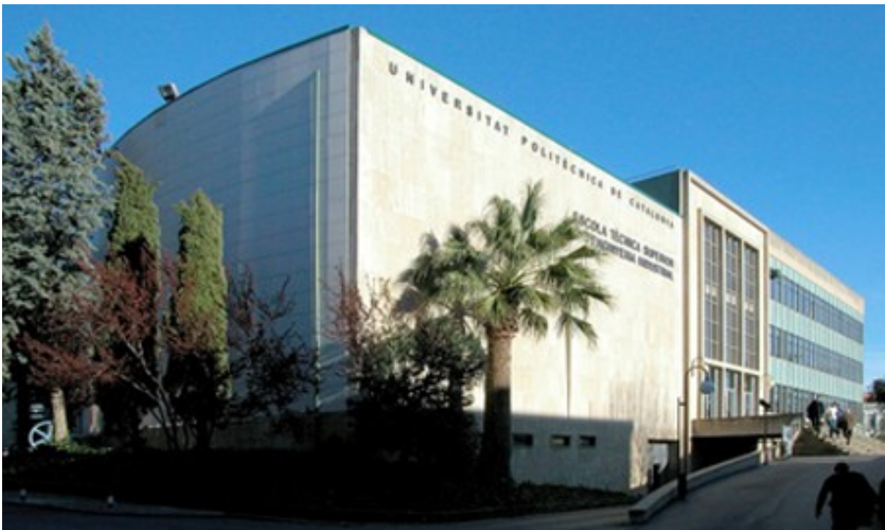
Figure 4.1: TR5 ESEIAAT building
