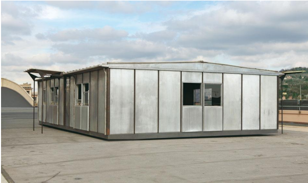
Images 75 and 76. Exterior and interior views showing the metal structure of the Maison Metropole.
