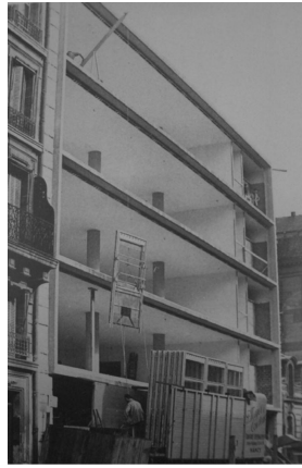
Images 83-84. Assembly of the panels in the FNB building from the inside.
