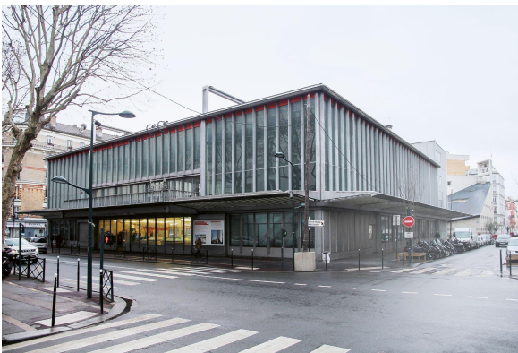
Images 73 and 74. Exterior and interior views showing the Vierendeel beams of the Maison du Peuple.
