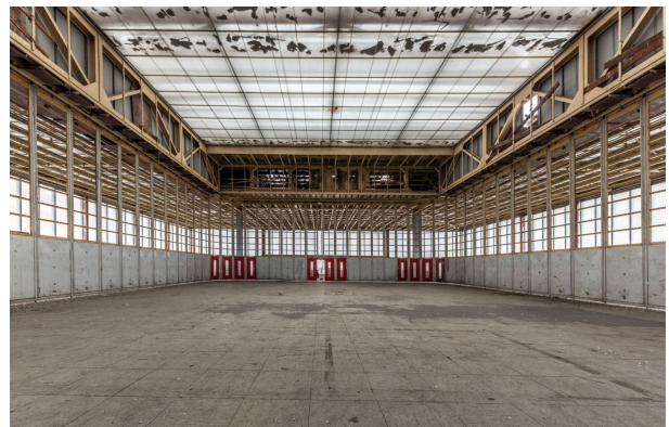
Images 73 and 74. Exterior and interior views showing the Vierendeel beams of the Maison du Peuple.
