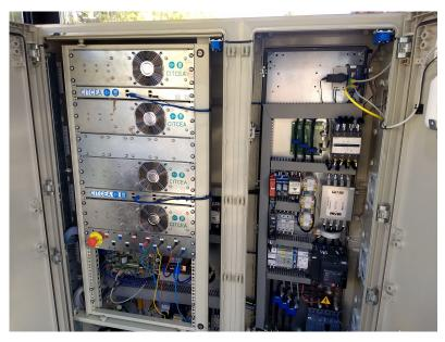
Figure 13. Detail of the Master Inverter power electronics.
