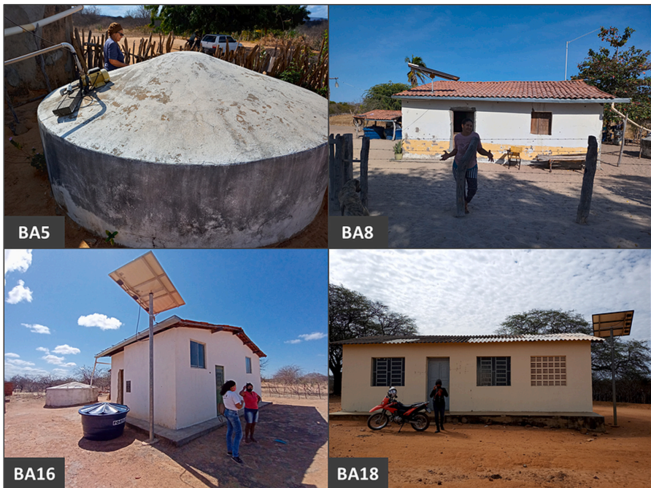
Fig. 3. Portrait of rural Bahian women. Two residential systems (13 kWh/month), powering the rainwater tank pump (BA5) and an external light point (BA8), and two community systems (30 kWh/month) installed in a production centre (BA16) and a school (BA18) are presented.
