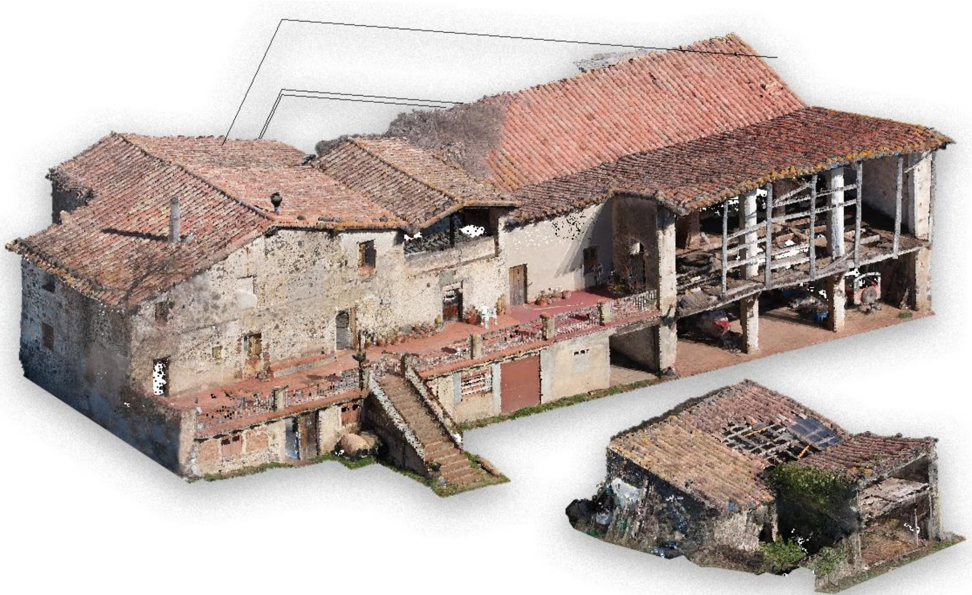
Vista de la geometria de Mas Maçandell amb model Revit. Font: D'autor. / View of the geometry of Mas Maçandell with Revit model. Source: From author.
