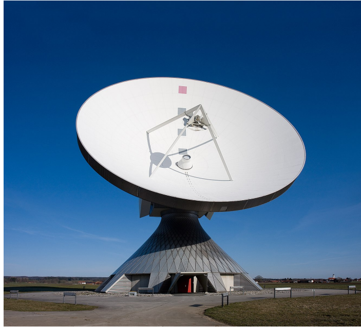
Figure 3.12: Parabolic reflector antenna.
