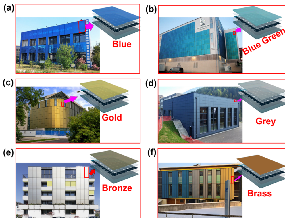
Figure 12. Kromatix™ technology-based PV modules and their applications. (a) Retrofitted building of Swiss Federal Institute of Technology of Lausanne (EPFL) with blue modules (reproduced and modified with permission from Ref. [109]), (b) blue-green BIPV wall made by the Swedish Research Institute (RISE) in Bors, Sweden (reproduced and modified with permission from Ref. [109]), (c) BIPV façade by gold PV panels of the Red River College Innovation Center, at Winnipeg, Canada (use with the permission; copyright. SolarLab.dk and Garry Kopelow) [110], (d) grey BIPV of the school gymnasium in Leysin, Switzerland (reproduced and modified with permission from Ref, [114]), (e) bronze colored BIPV façade in a residential building in Zurich, Switzerland (reproduced and modified with permission from Ref. [102]), and (f) Doma Solartechnik Headquarters in Satteins, Austria (reproduced and modified with permission from Ref. [116]).
