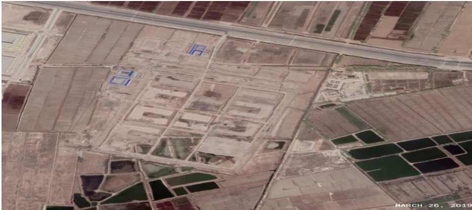
Figure 6g: Shufu county, Xinjiang detention facility showing the site location for housing 10,000 forced workers. Satellite image date: March 26, 2019. Source: (Rajagopalan and Killing, Alison; Buschek, 2020).
