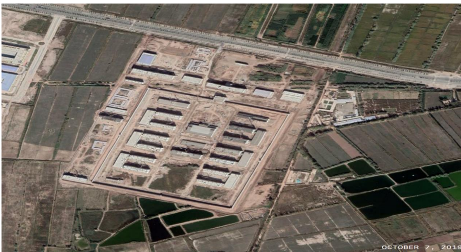
Figure 6h: above Shufu county, Xinjiang detention facility showing considerable progress in construction development over a period of less than 7 months. The facility is meant to house 10,000 forced workers. Satellite image date: October 7, 2019.
