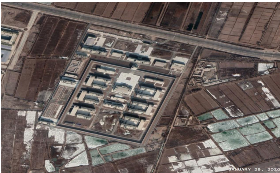
Figure 6i: Shufu county, Xinjiang detention facility showing full completion over a period of 10 months. The facility is ready to house the intended 10,000 forced workers. Satellite image date: January 29, 2020.
