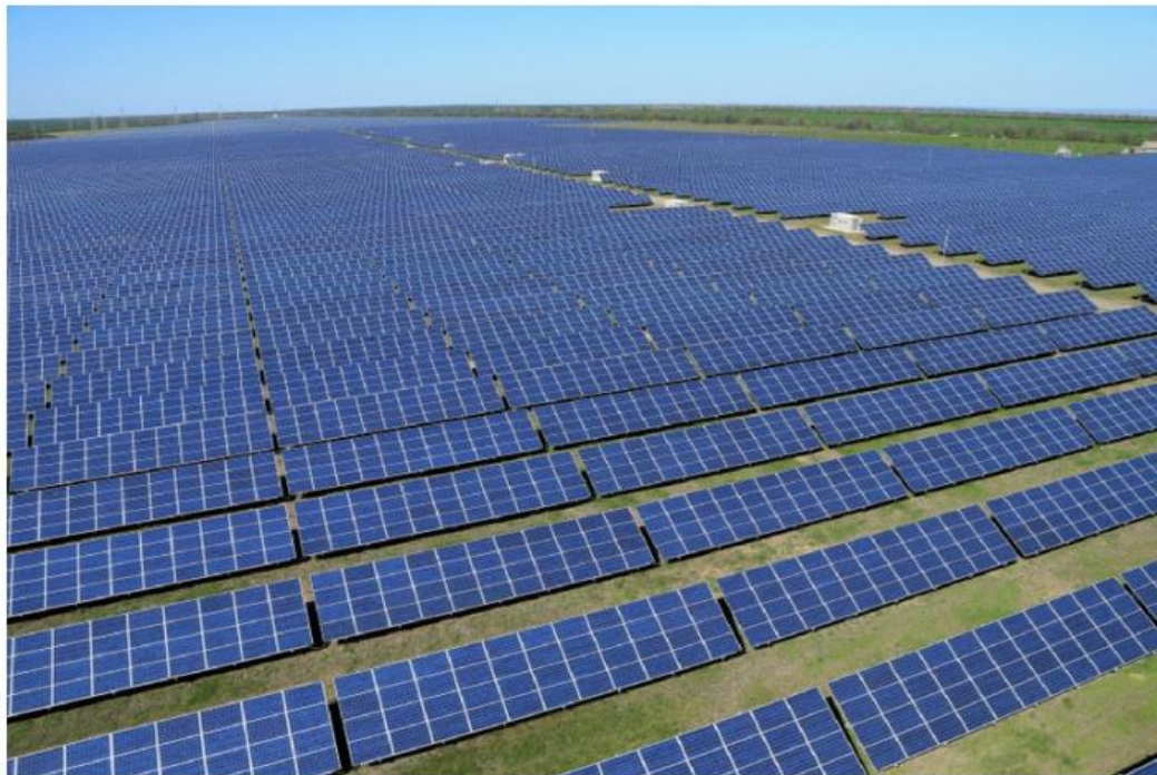
Figure 7k: Bhadla Solar Power Plant, Rajasthan (2245 MW). Source: (Prateek, 2018).
