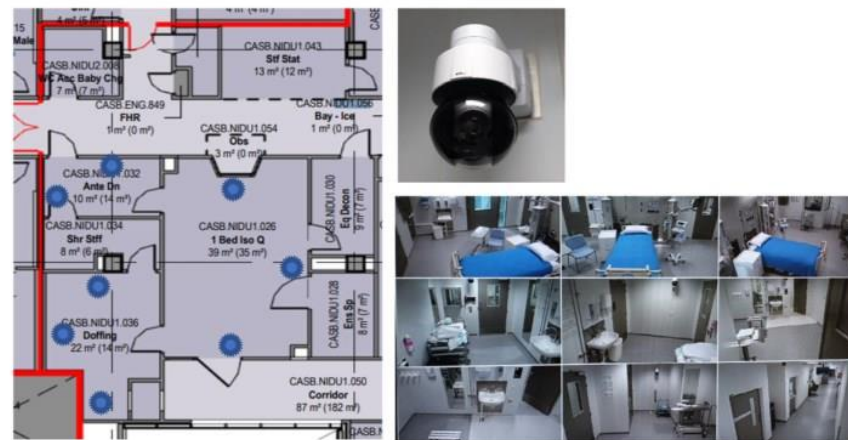
Fig. 1. Camera system in place in the NSW Biocontainment Unit; placement of cameras, close up image of camera and sample of camera field of view.
