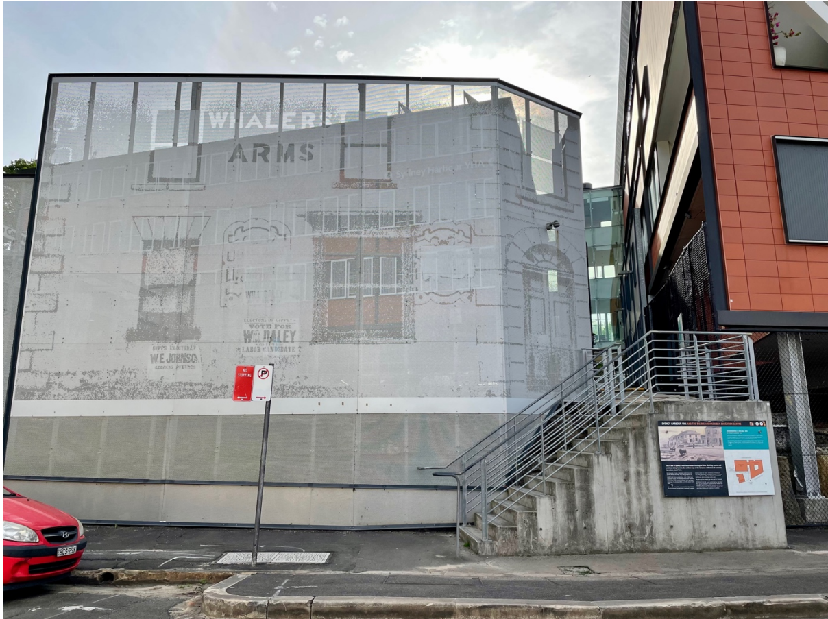
Figure 4.7: The Exterior of the Sydney Harbour YHA from Gloucester Street showing the interpretive screens designed to evoke the facades of the buildings that stood on the site in the nineteenth century (Image Credit: Caitlin Allen 2019).
