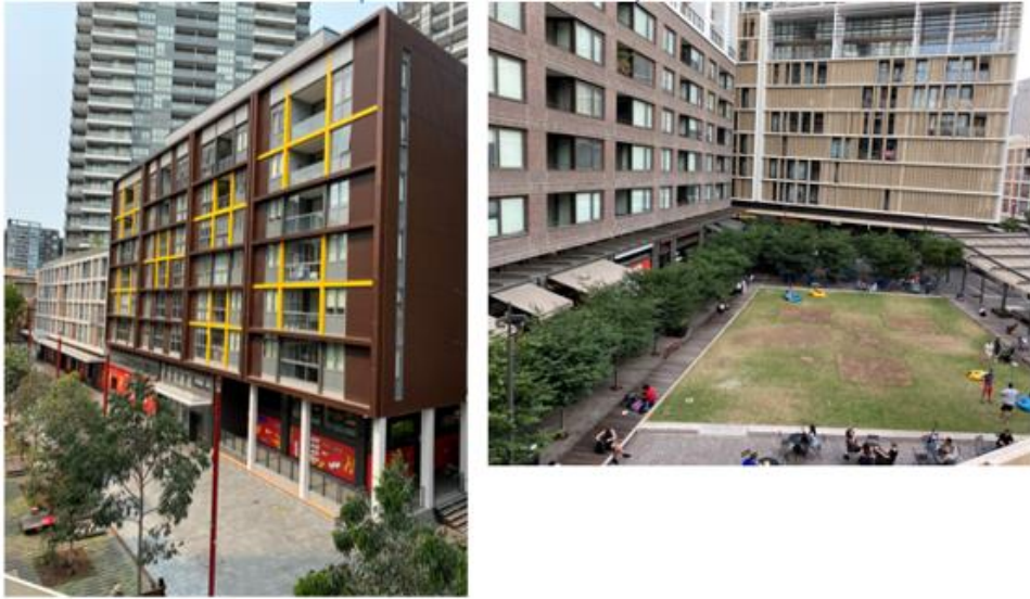
Figure 42. Photos: Eldridge, T, Patterns of the building facades with both varied and monotonous designs, Darling Square, 15/1/20.
