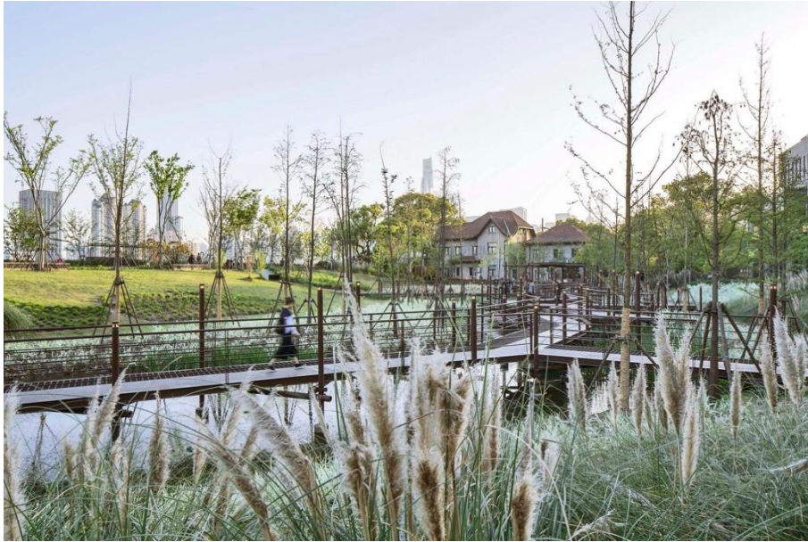
Figure-5. The steel corridor bridge across the wetland 26)
