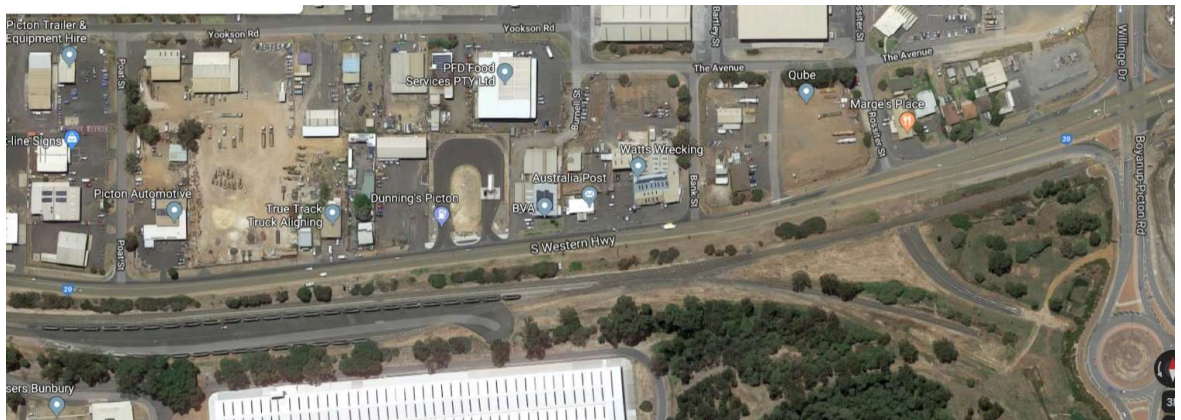
Figure 7-22 - Picton rail siding.
