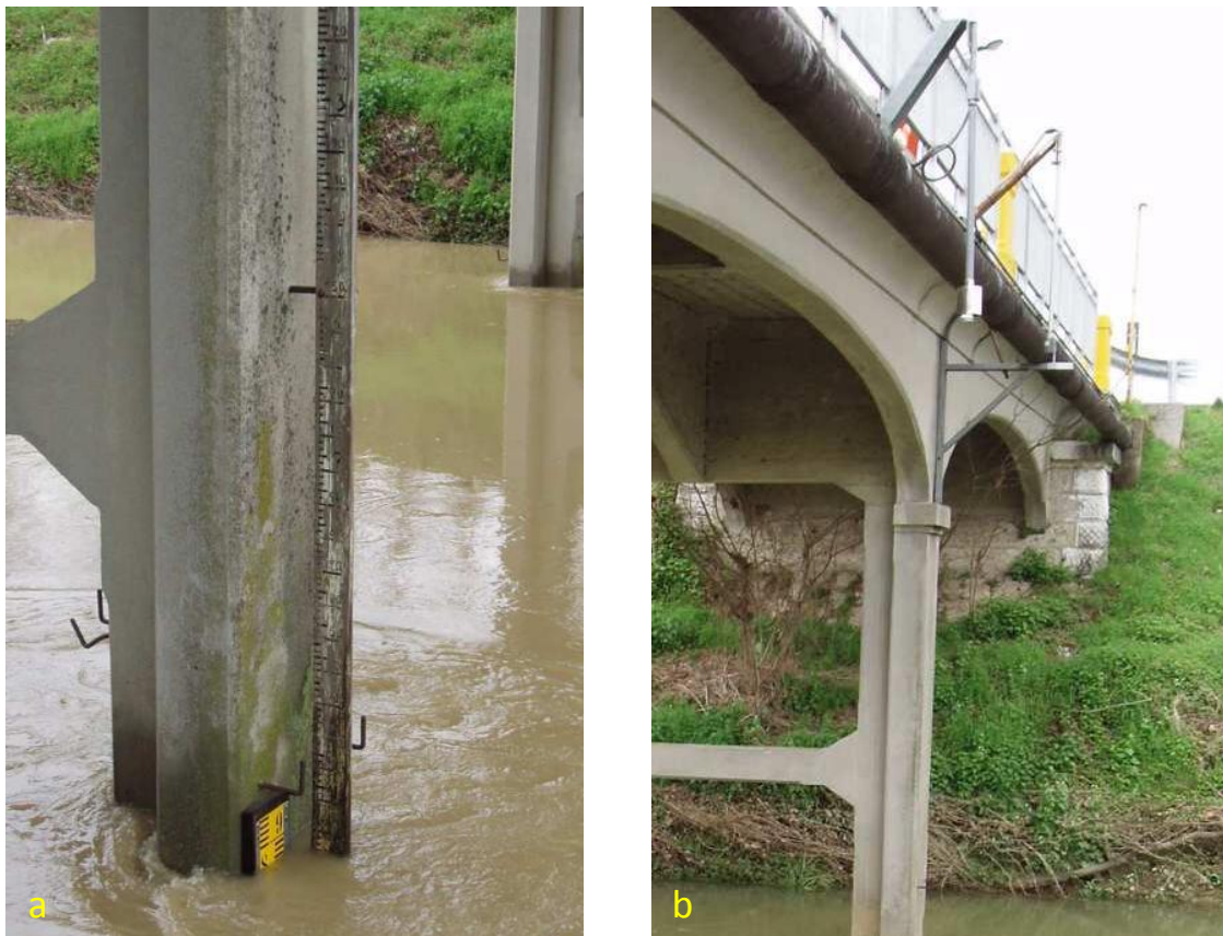
Figure 3.6. a) Hydrometric rod and b) Tele-hydrometer at Fontanelle station
