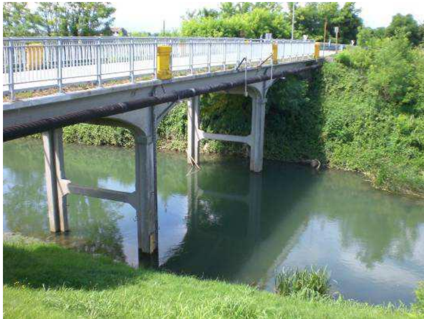
Figure 3.5. Hydrometric level measuring at Fontanelle station
