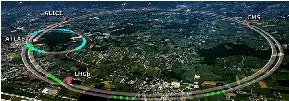
Figure 3.2: Panoramic view of the area occupied by the Large Hadron Collider ring.
