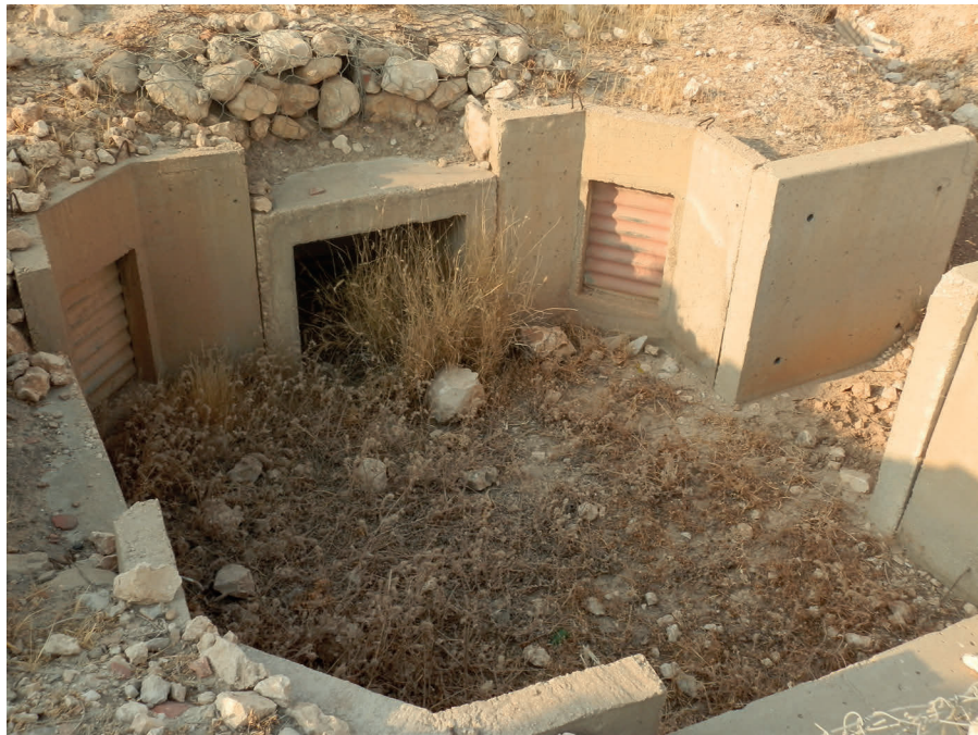
FIGURE 3 Khirbet el-Makhruk, Jordan valley: firing position in concrete built directly on Iron Age remains (original picture taken by the author in 2012)
