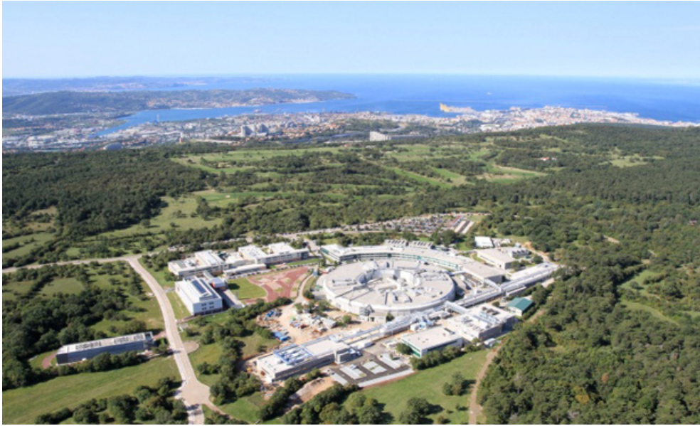
Figure 2.2: The Elettra Synchrotron Radiation and Free Electron Laser Facility in Trieste. Panoramic view [21].
