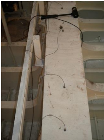
Figure 48 - measurement points on a diesel engine foundation
