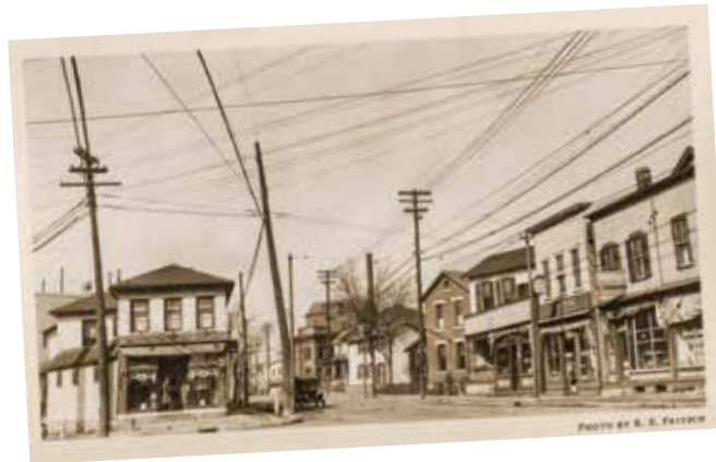
WIRES CRISSCROSSING ON BROWN STREET, AT WARREN STREET, LOOKING NORTH.
