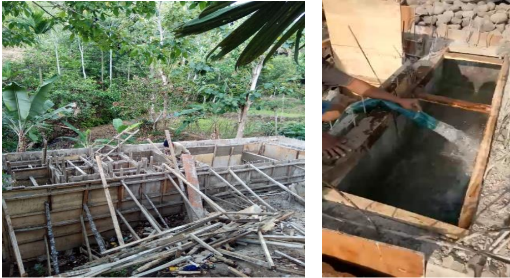
Figure 4. Wastewater Management Construction of Batuputuk and Langkapura Baru
