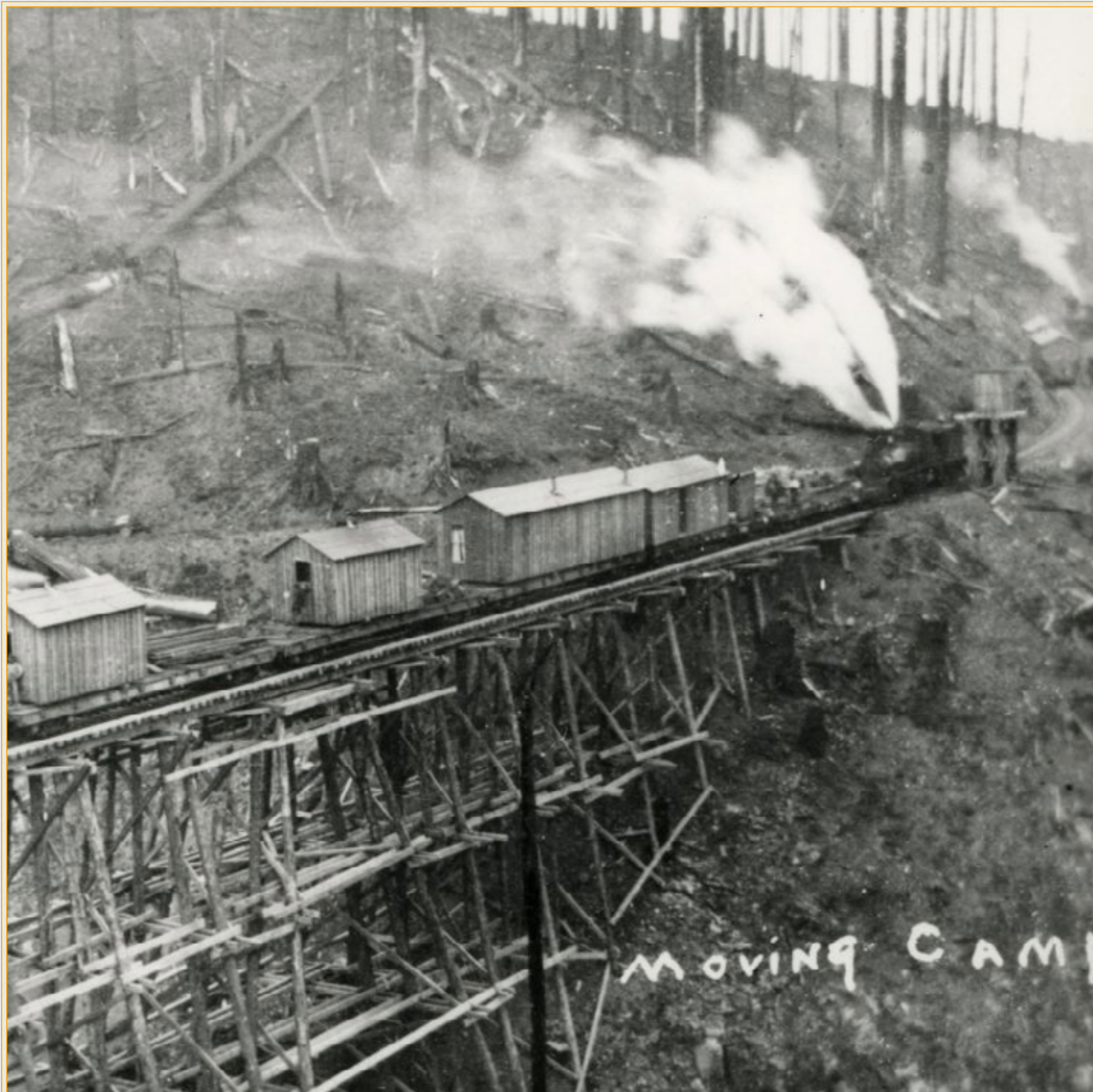
A train hauls timber camp buildings across a trestle in the woods on the way to the next harvesting site.. Courtesy Oreg. Hist. Soc. Research Lib., OrHi48497 Large Wood, Long Legacy
