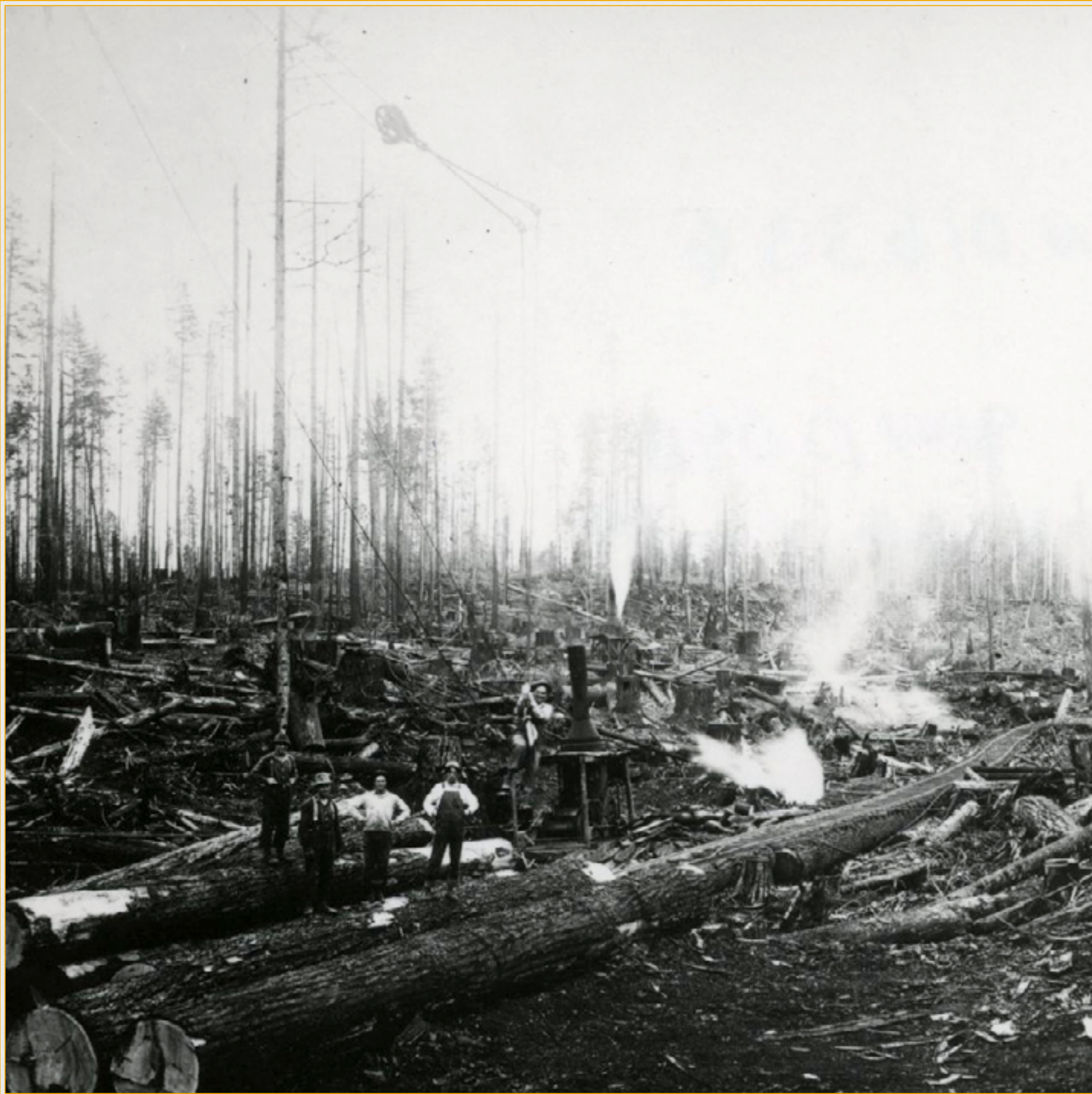
Men stand near four donkey engines at work in a clearcut, Pacific Northwest. Courtesy Oreg. Hist. Soc. Research Lib., 016336 Large Wood, Long Legacy
